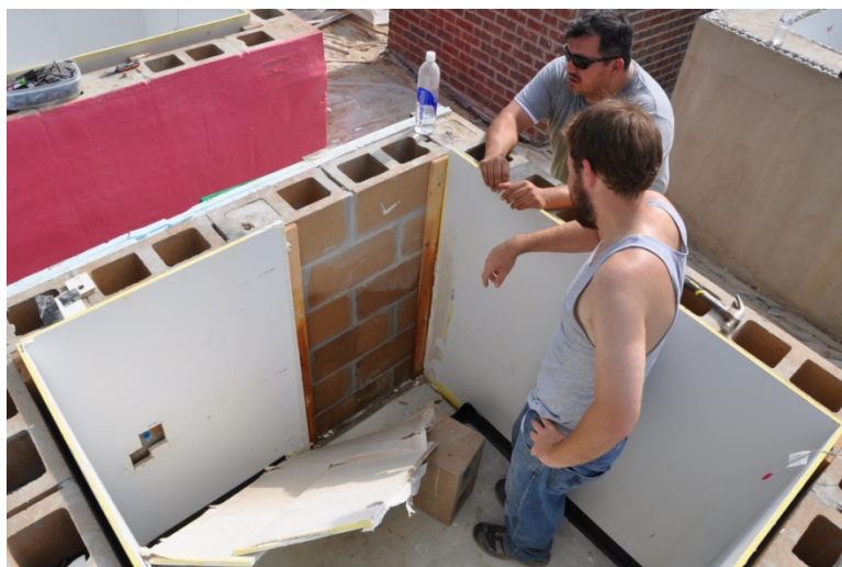
Fig. 4.5. PHOTO: Partial demolition of test pod after flood simulation 1.
